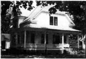
65 201 Clark Street, Birkholz House (Raymond Havey House): Built in 1907. The house is of transitional style incorporating Queen Anne features (such as the scalloped shingles on the gables) and Colonial Revival motif (such as the full-width front porch). The builder was a contractor by the name of Grosholtz. The house is in an excellent state of preservation.
