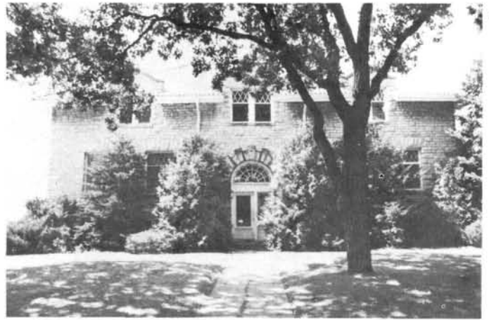
Main Entrance (East facade) of office building today.
