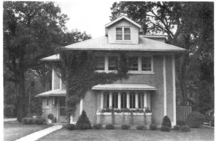
49 106 Blunt Street, George Blake House (Richard Austin House): Circa 1913; a Prairie School house, in good condition, with panelized walls of stucco, decorative tile insets, broad overhanging hip roof, and "banding" of windows. The dormers added in 1951 mar the original design. The architect was Morton B. Cleveland of Waterloo, Iowa.
