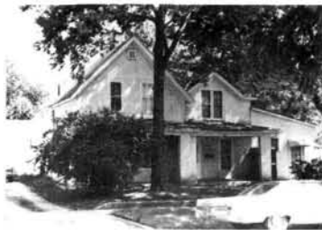
106 N. Iowa Street, Richard Miles Waller Cabin (Don Molitor Building): Circa 1855. The north, two-story portion of this building is a log cabin which was the first home of R. Miles Waller, one of the developers of Charles City. The log walls were covered over with stucco upon expansion and the addition of a porch. A frame, shed-roof addition, wrapping around two sides of the earlier buildings and a "barn", at the rear of the lot, were subsequently constructed. The property, generally in fair condition, is used for commercial as well as residential uses.
