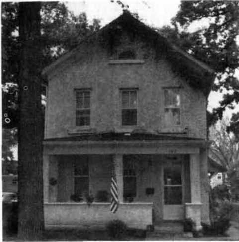
37 102 Ferguson Street, Kannengeiser House (Bernard Faught House): Circa 1865; a simply styled house of local limestone and long covered over with stucco. The attic window is fan-shaped. In good condition, the house has undergone interior alterations including removal of some interior walls.
