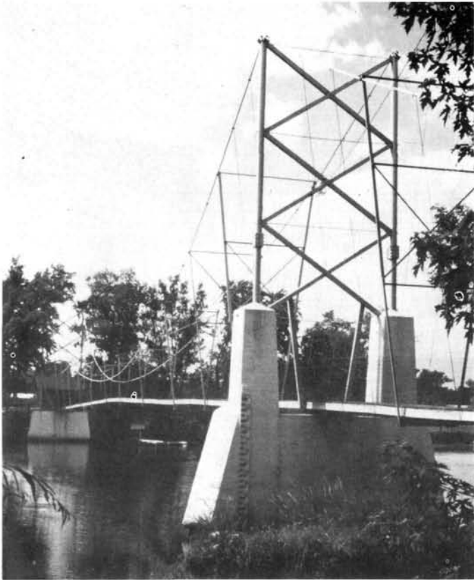
View of Foot Bridge, circa 1906, showing supporting steel posts for the steel suspension cables. Post card view from Lee Albaugh collection.
