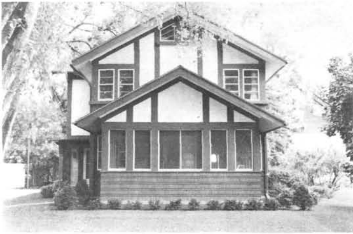
48 104 Blunt Street, historic name not identified (James Willeke House): Circa 1918; a Prairie School house, in excellent state of preservation, with broad overhanging roofs and use of natural materials. The walls are articulated with stucco panels set off by wood trim and pentagonal gable windows.
