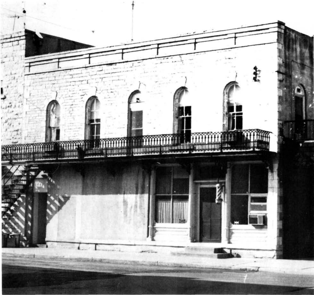
Addition built in 1877 to the 1863 Gilbert's Stone Block/Union House (identification no. 5).
