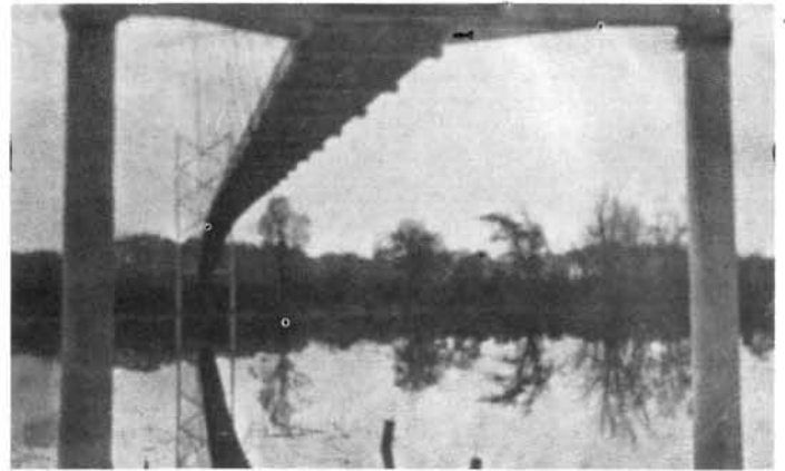
View of Foot Bridge, circa 1906, showing supporting steel posts for the steel suspension cables. Post card view from Lee Albaugh collection.
