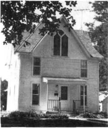
91 1414 Clark Street, J. Mall House (C. Miller House): Circa 1885; representative of "budget" Queen Anne style of the period. The house, in fair condition, has gables of various patterned shingles and the window of the front gable is a unique combination of paired pointed windows with a rotated square window accent.
