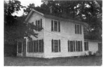
306 Blunt Street, Ellis House (Henry Emmel House): Circa 1860; a simply styled house, in fair condition, with small-paned narrow windows and turned porch posts. Decorative wood strips suggesting shutters are a recent application.
