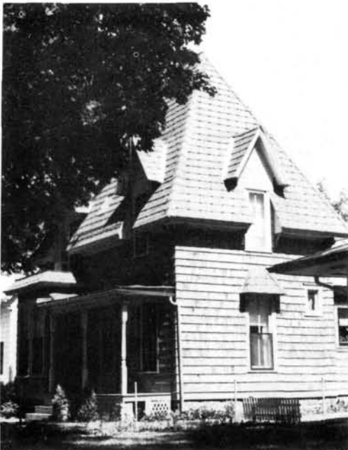
1515 Clark Street, R. T. Roethke House (Sylvan George House): Circa 1885; a unique house with steeply pitched hip roof. The house, in fair condition, is handsomely textured with shingles on the walls and roof; essentially, it is of Queen Anne style with carryovers of the Gothic Revival.
