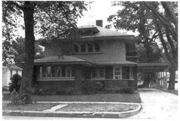
47 103 Blunt Street, Smith House (Methodist Parsonage): Built in 1914; a well-preserved house with Prairie School influence; wide overhanging hip roof, horizontal lines, grouping of windows, stucco over brick. Only the dormer and attached carport addition detract from the design. The builder was Guiwits; the architect was probably Morton B. Cleveland.
